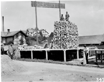
Photo: ETH-Bibliothek Zürich, Bildarchiv, Slab and beam tests, Joistless ceilings (mushroom ceilings), 1908
